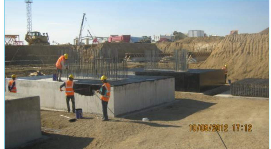
Concentrator building foundations, first concrete
