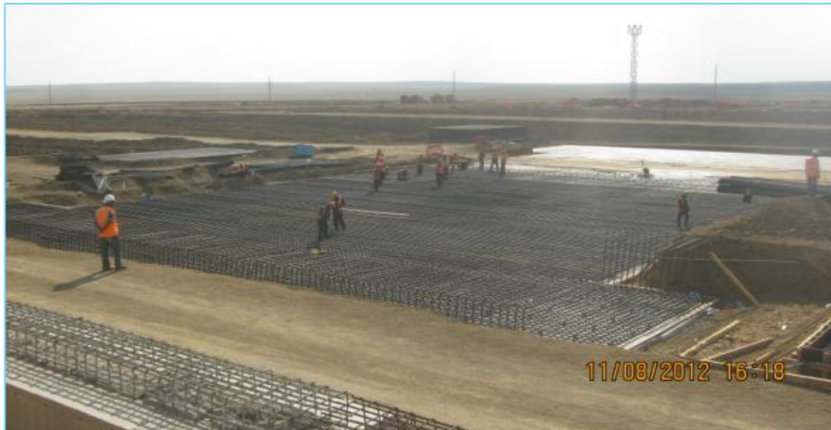
Rebar fixing for ball mill foundation
