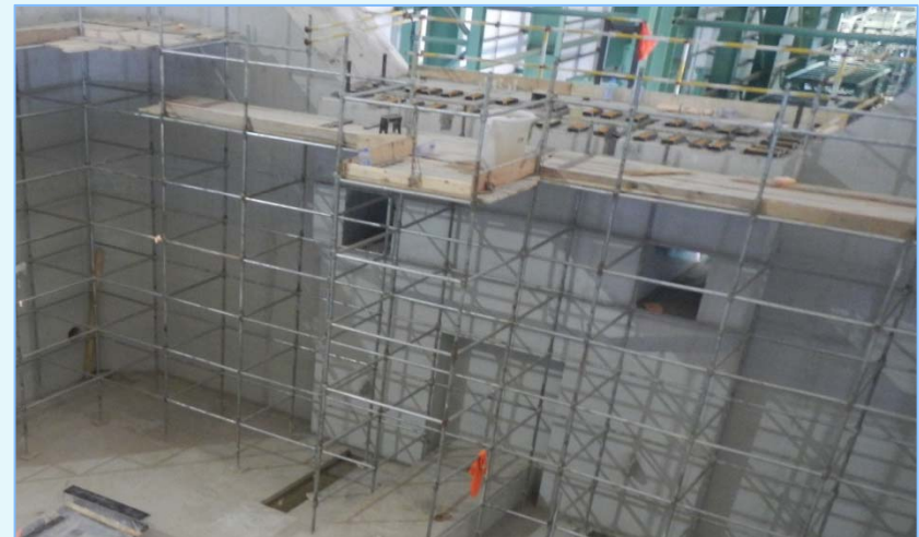
Installation of sole plates for SAG Mill
