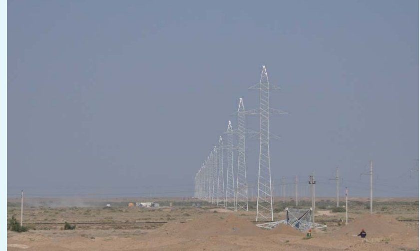
110 kV power line (50% complete)
