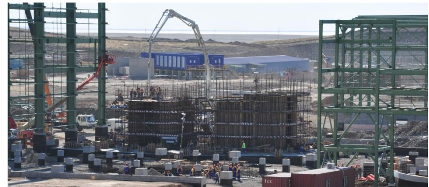
Flotation and regrind area, foundations and steelworks
