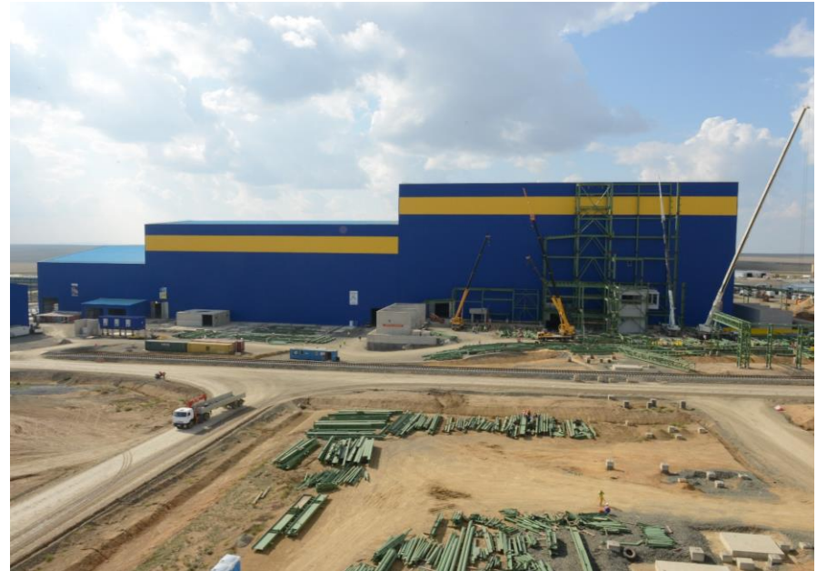
Bozshakol concentrator construction, 2014
